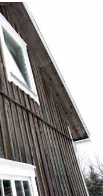
• The panelling was treated with copperas and then put to lie outdoors for a year, just to get the right shade of grey.
