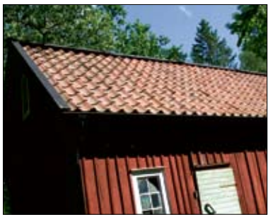
The first try with ridges of solid wood shows that the product stands the test.
