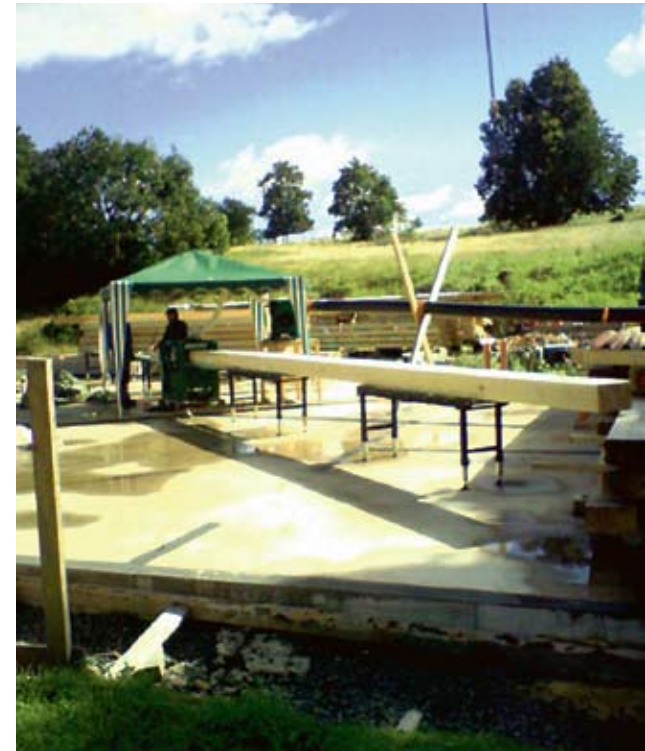
This is the photo that Per-Arne took with his cellphone, showing the planing of a 12 metre long beam with the measurements 8" x 12".
