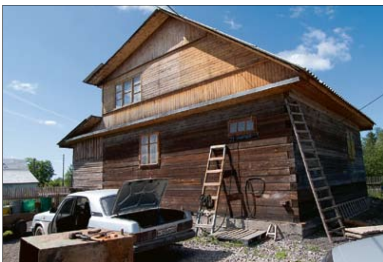
The house Andrej had begun to build when the old sawmill disappeared.
