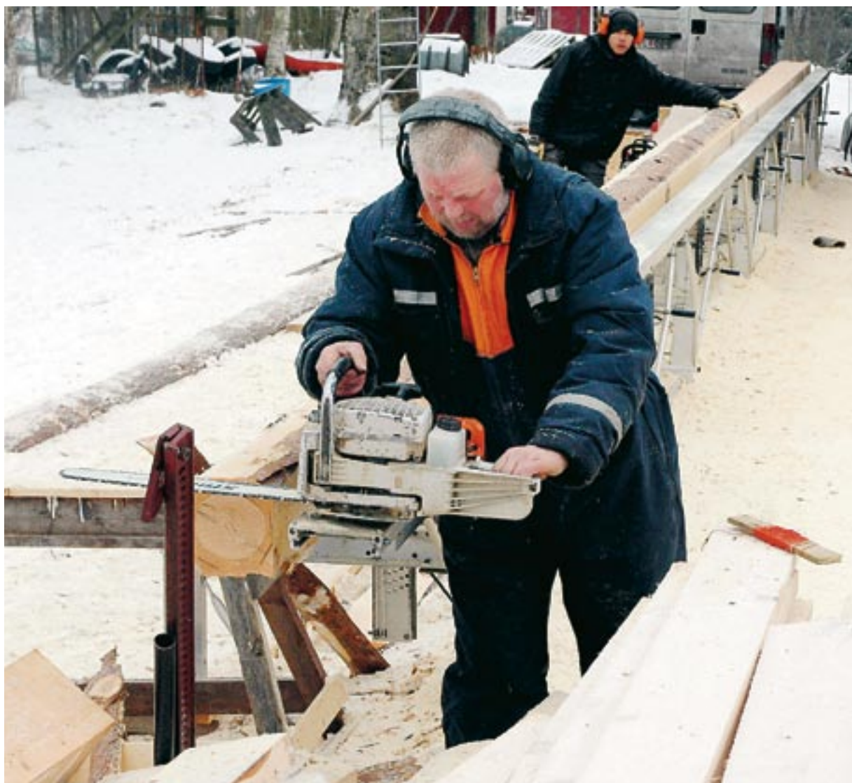
Poul Nielsens three and a half M7s were the only way that the 17-metre long, ruler straight beams could be cut out for use in rebuilding the church tower in Vadensjö.
