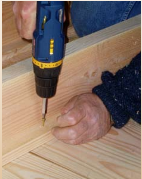
The T-beams are screwed to the bottom.
