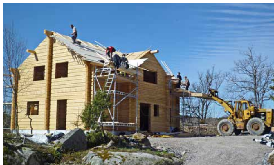
• During spring 2012, the timber frame was erected and the house got its roof of self-made T & G boards.
