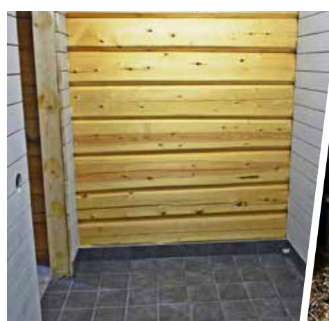
• During 2013 the laundry room was completed in the new house, in order to get the heating system started. They chose nice tiles and wooden walls that were planed with knives that give a rougher surface.
