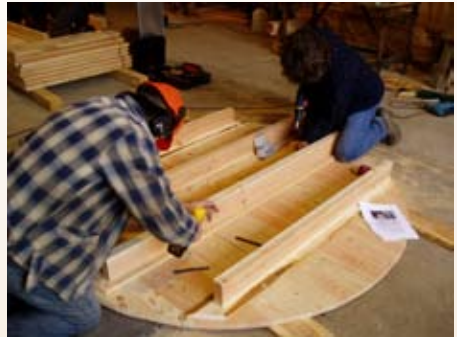
The T-beams are screwed to the bottom.
