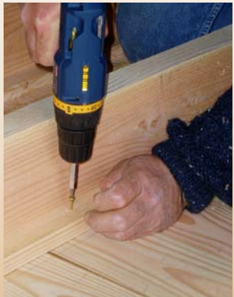
The T-beams are screwed to the bottom.
