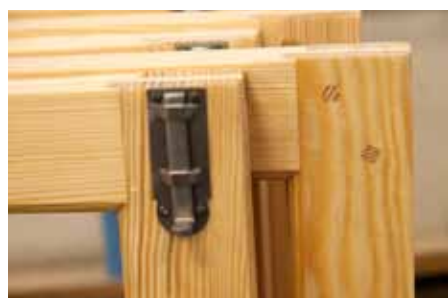
• The window frames are put together with wood dowels to make it easier to replace damaged details in the future.
