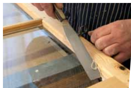
• The window frames are put together with wood dowels to make it easier to replace damaged details in the future.
