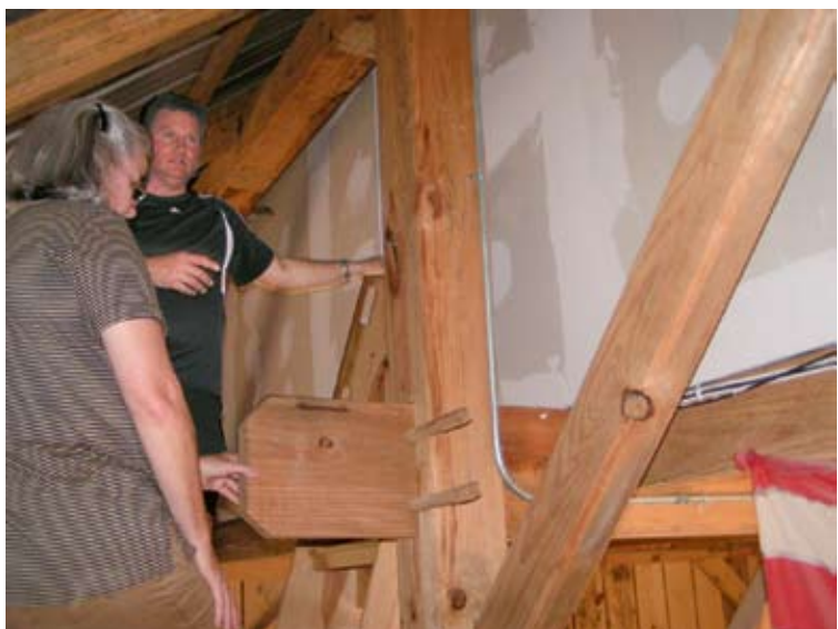
Greg shows Kathleen Griffin some of the details of the joinery that went into the barn. All framing members are held together with wood pegs.
