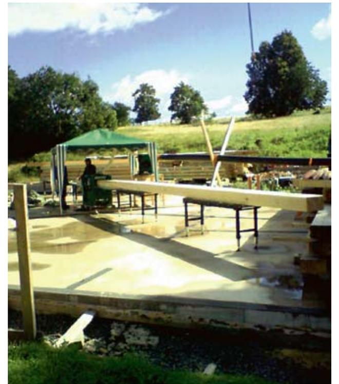
*This is the photo that Per-Arne took with his cellphone, showing the planing of a 12 metre long beam with the measurements 8" x 12".*
