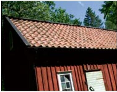
The first try with ridges of solid wood shows that the product stands the test.
