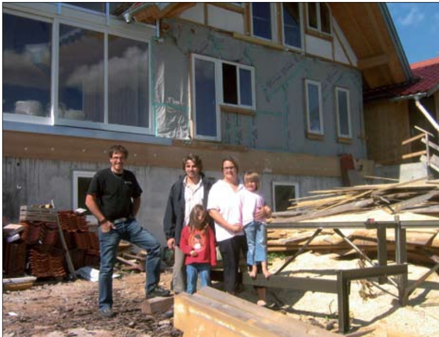
BUILT A NEW HOUSE AFTER THE STORM! After a big storm in Germany the Pfeifle family built the house of their dreams. Don't miss their story in the Logosol e-newsletter!
