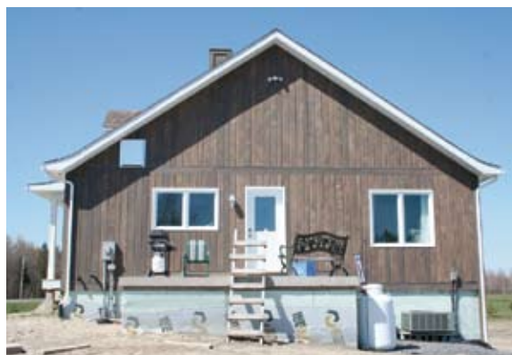
The White Pine siding is produced with the 4-sided PH 260 planer moulder.
