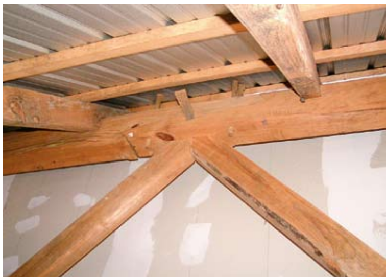
Greg shows Kathleen Griffin some of the details of the joinery that went into the barn. All framing members are held together with wood pegs.
