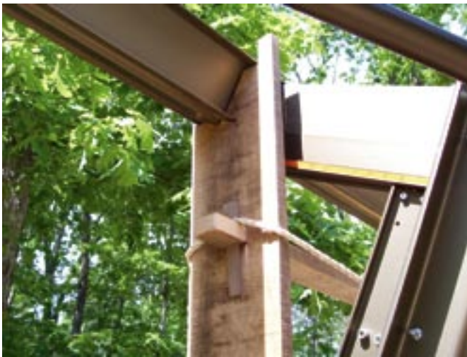
Ailanthus wood has large pores and is 'rough-grained.'
