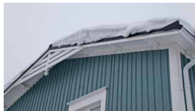
• Profiled support brackets and moderate gingerbread work embellish the gable ends.
