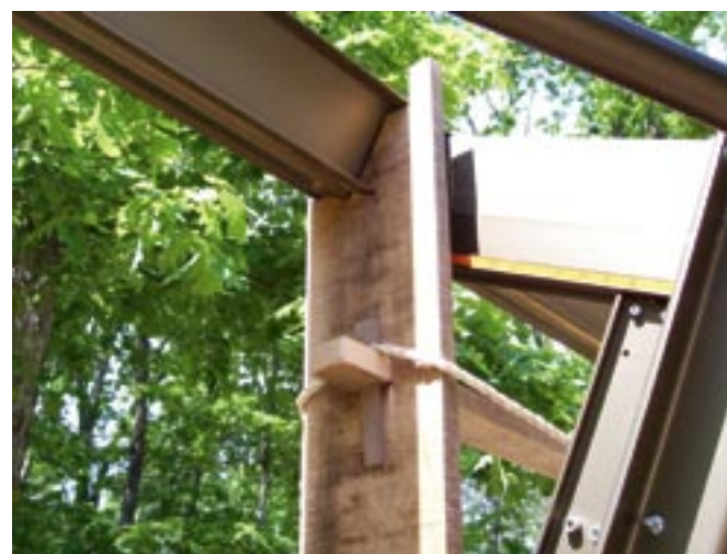
Close-up of wedged through-tenon holding top of carrying rack.
