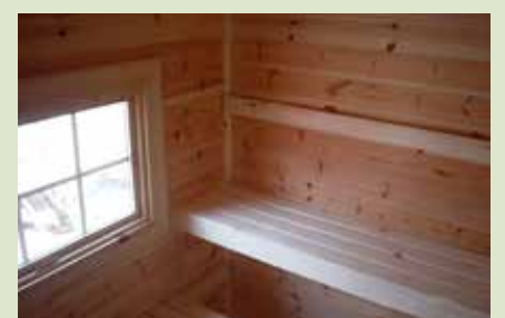
• Benches of aspen in the sauna cabin, which comes fully built of dovetailed planks.
