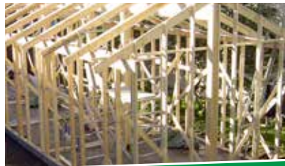
JOISTS FOR THE FRAMEWORK
