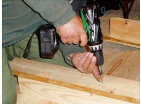
The T-beams are screwed together.
