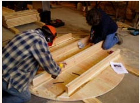
The T-beams are screwed to the bottom.
