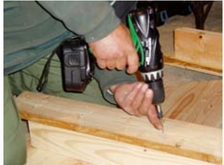
The T-beams are screwed together.
